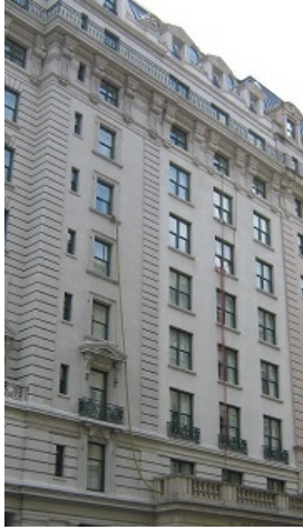
ePIPE was used to restore this hotel's potable hot water system
