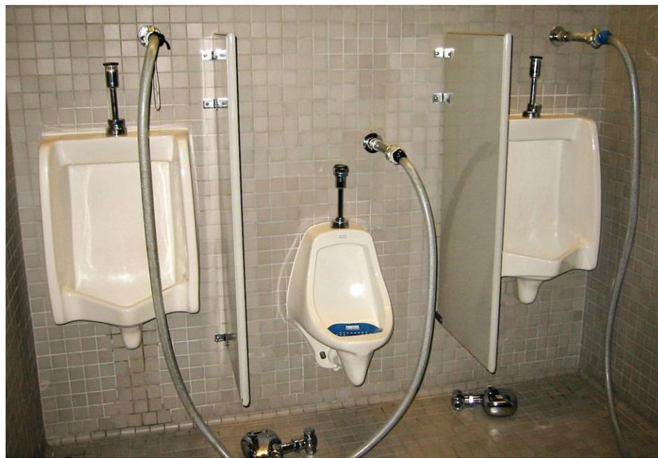
Pipe-lining technologies such as ePIPE, used in this picture, reduces disruptions to normal business activity in commercial properties.
